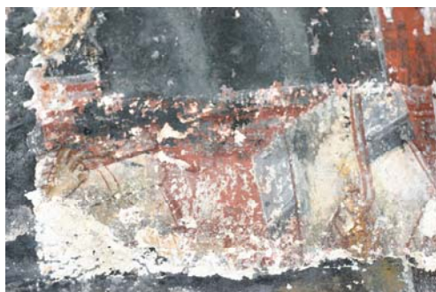
Fig. 2. Details of the two layers of paint from the 17 th (middle layer) and from the 19 th century (upper and lower layers) from one of the walls in Sv. Bogorodica Church in Lešok. (The colour can be seen on the on line Internet issue)
